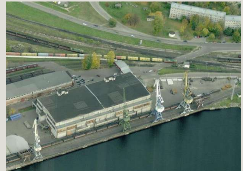
A view to the former warehouse building at Eksporta iela 15 k-8, behind it there is a building at Eksporta iela 15 k-9
